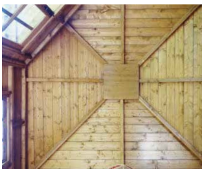
Internal roof structure
