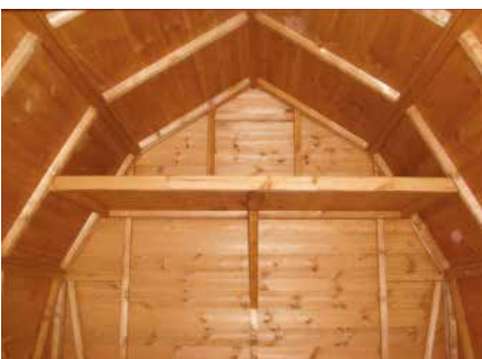
Internal roof and shelf
